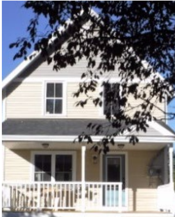
59 Baxter Street, Rutland Neighborhood & Housing Revitalization
